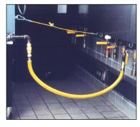
**WARNING:** Per the ANSI Z21.69 / CSA 6.16 Standard, Gas Connectors cannot be reused when an appliance is being replaced or moved to a new location.
